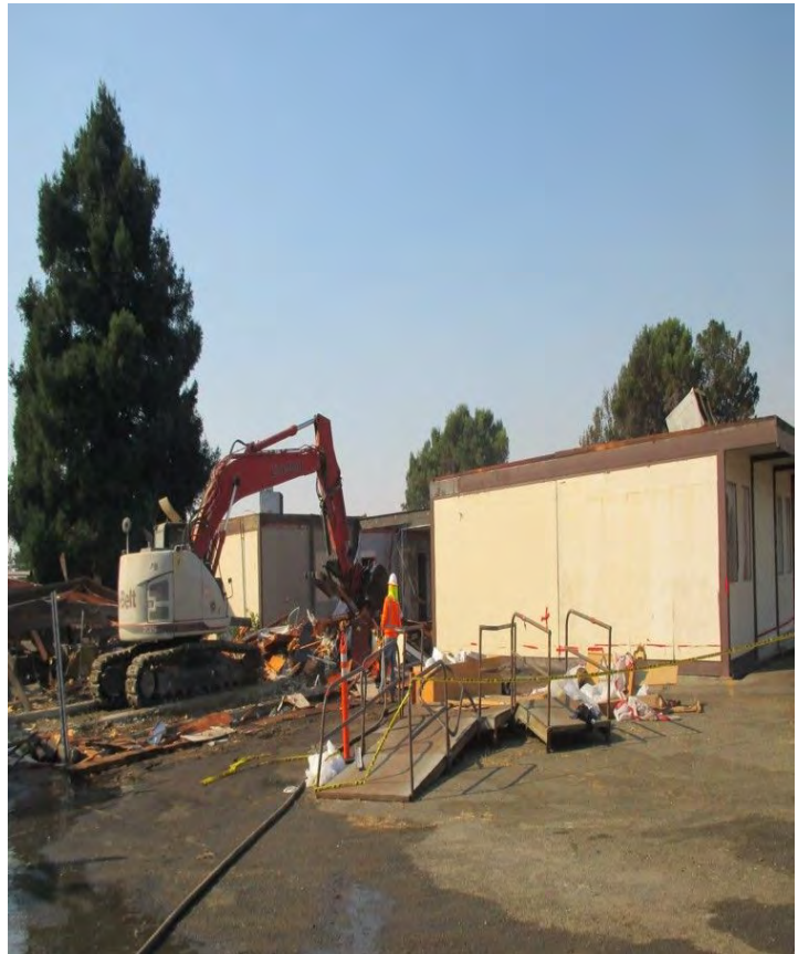
Harmon Knolls Demolition
