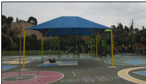
Valley View Elementary School
