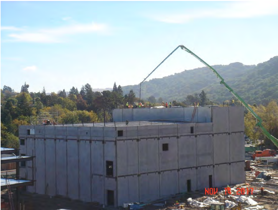
Pinole Valley High School - Performing Arts Building
